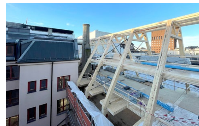
At the top of the building at Øvre Vollgate 11, two new floors are being built in glulam from Moelven.
